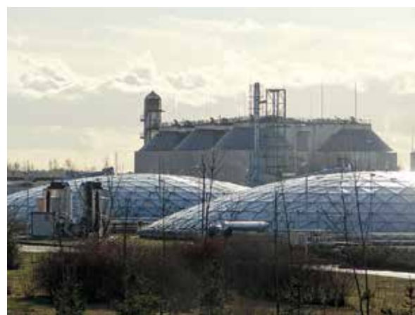
Figure 2. Wastewater treatment plant in Koziegłowy, Greater Poland district, Poland. The sludge tanks are now, after a lengthy print and electronic media campaign, covered with protective domes to reduce the malodor and prevent environmental mishaps
